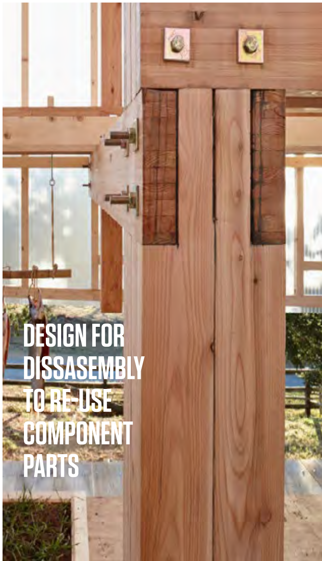
© Kengo Kumma & Associates + College of Environmental Design UC Berkeley / Shinkenchiku Sha
